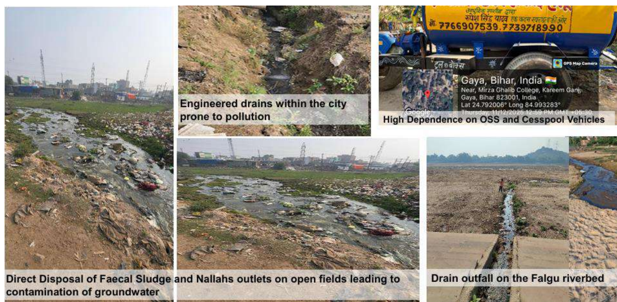
Figure 21: Sewage network issues
