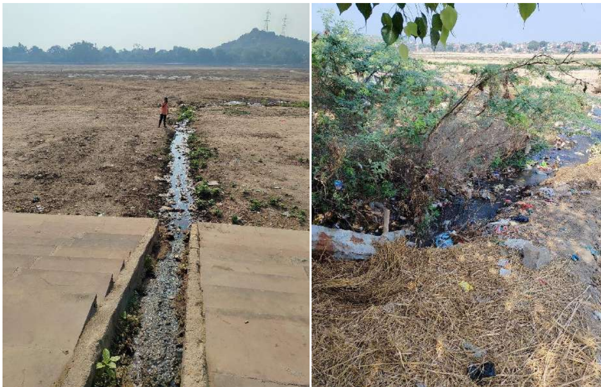
Figure 33: Discharge of Untreated Wastewater in the Water Body – Falgu River
