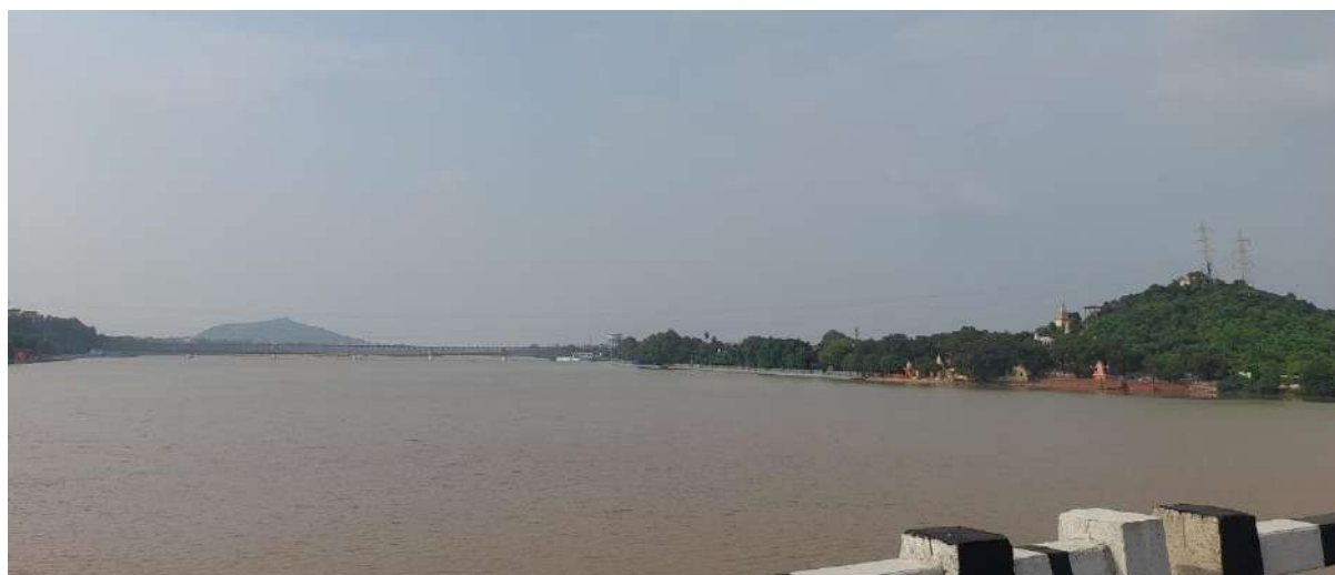
Figure 47: Distance View of Concretisation of the Bank along Falgu River on Manpur side
